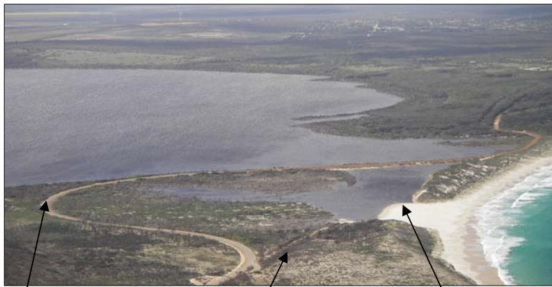
Hamersley Drive crossing Culham Inlet, (photo by Mieke Bourne, 2007)
